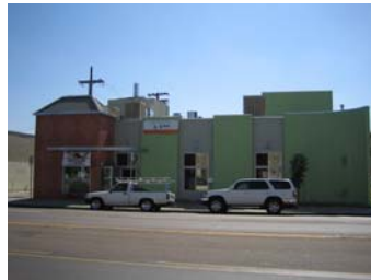
Tortilleria Lily is the first renovation to be completed under Adopt-a-Block.
